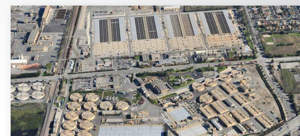
Joint Water Pollution Control Plant (JWPCP)
