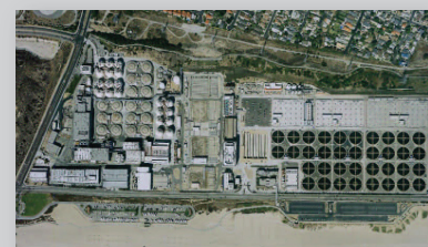
Hyperion Treatment Plant (HTP)
